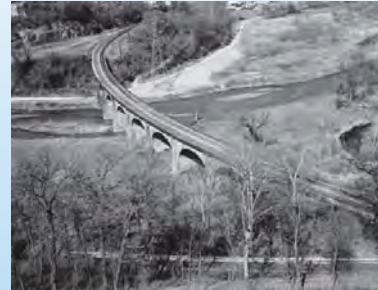
B&O Railroad Thomas Viaduct
